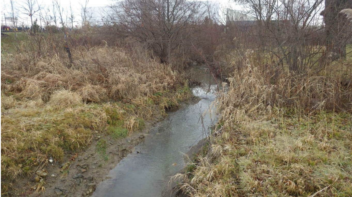
Photograph 49 Haines Ditch facing east (upstream) from the Beech Road Culvert. (EMH&T, 12/17/2021)
