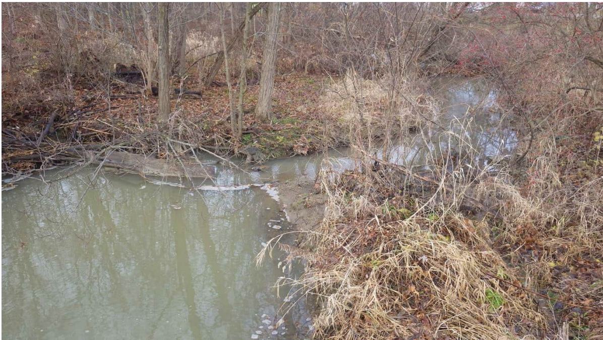
Photograph 50 Haines Ditch facing west (downstream) from the Beech Road Culvert. (EMH&T, 12/17/2021)
